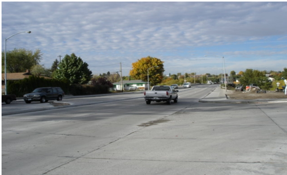
Greene Street looking north from Spokane Community College after completion of construction.
