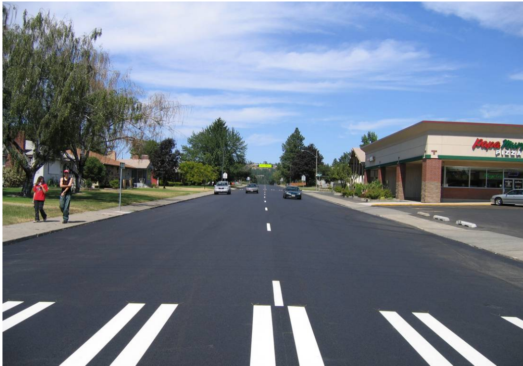
Southbound Ash Street just north of Rowan Avenue after completion of construction.
